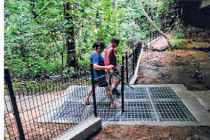
Above: Signage at Zhenhua Nature Park reminding visitors of the dangers of encountering a wild boar. Left: The Bangkit Underpass features a mix of fence and cattle grids which will deter wild boars from crossing, while allowing access to park users and cyclists. ST PHOTO: LIM JIE
