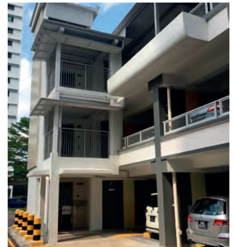
Lift installation at multi-storey carpark
