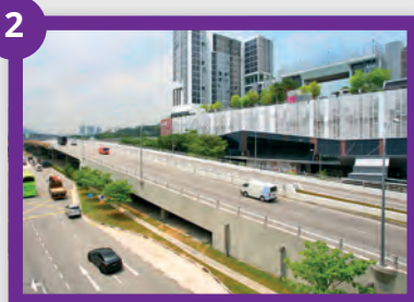
Bukit Panjang Flyover: Smoother Traffic, More Convenience
