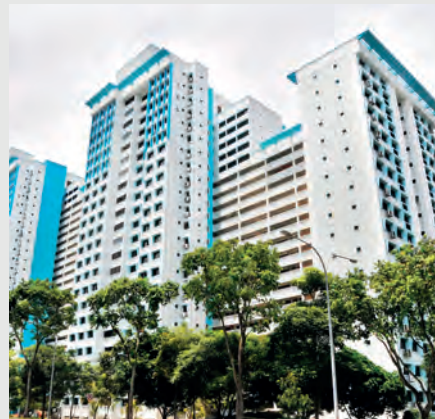
Petir Road – Repainting and Repair
